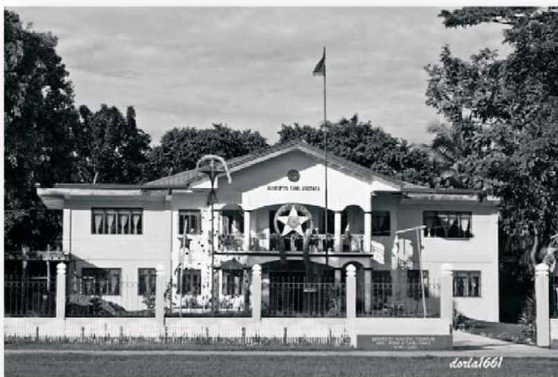
Municipal Building, Agutaya
